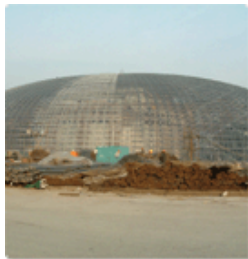
Grand National Theater (Under construction)
