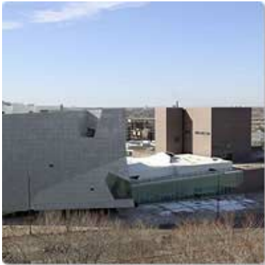
Walker Art Center, 2005. Herzog & de Meuron expansion (Theater Tower) on left and Barnes building (Gallery Tower) on right. February 2005 - a few months before grand opening.
