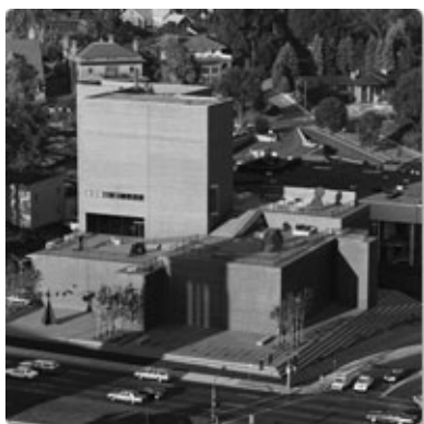
Barnes building in 1985; viewed from east. (The Guthrie Theater is building connected at right of Barnes with the banners extending from roof.)
