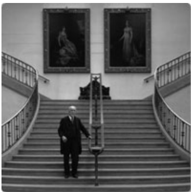
Photograph of TB Walker on grand stairway in the foyer of the newly-constructed Walker Art Galleries, 1927.
